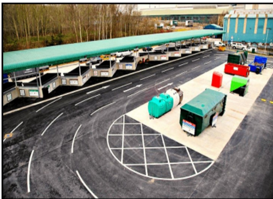
Cheadle Ave Household Waste Recycling Centre, Old Swan
